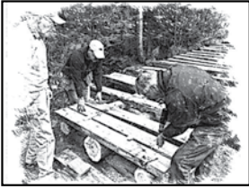
PBT Bridge Construction
