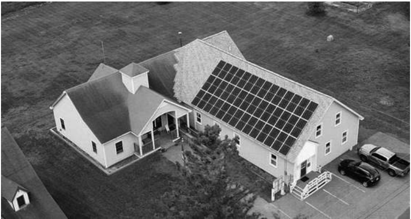
(Photo Provided by Sean Carlson of 603 Solar)
